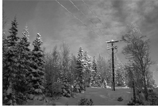
Distribution line with no ground wire.
