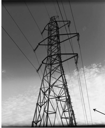
Distribution line with no ground wire.
