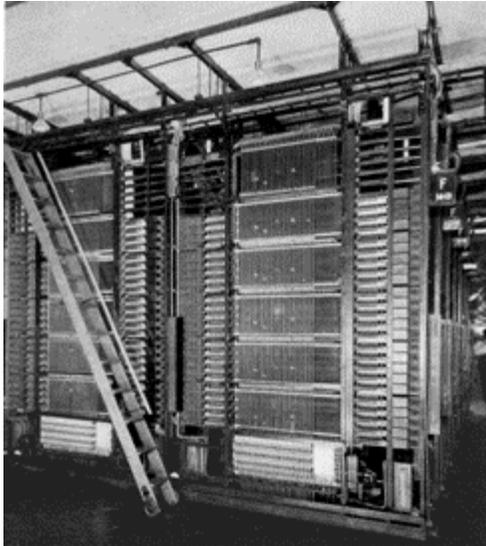
In 1921 the Bell System introduced the first commercial panel switch, an odd beast if there ever was one. Developed over eight years, it was AT&T's response to the step by
